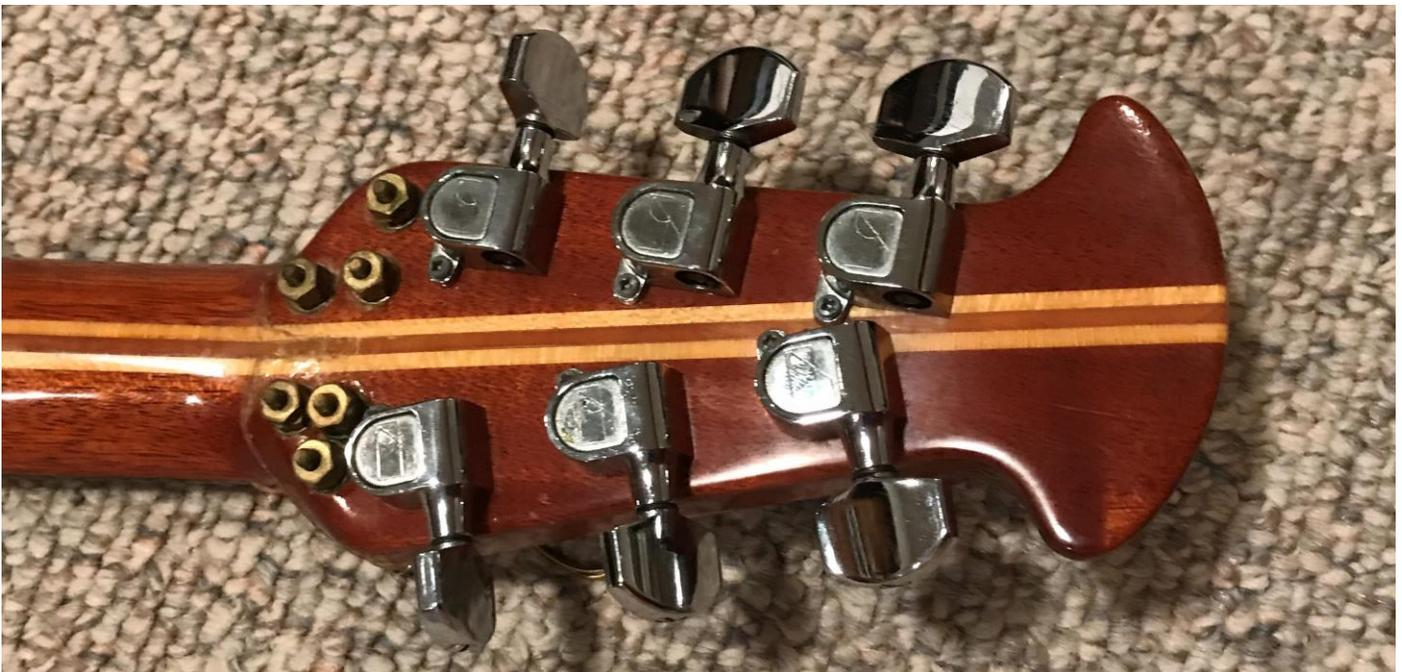
It never occurred to me to seek out a luthier that might have affected a nearly invisible repair. Instead I repaired it myself and you can see the result. The outcome was a fully functional guitar with an ugly head. The screws are the obvious part of the repair but I also used common wood glue.
